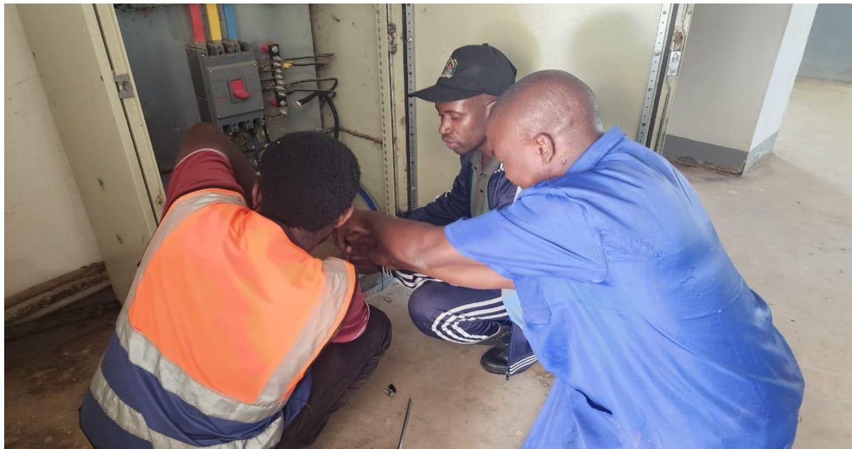
Image 1: Technical team together with St. Francis Ifakara Mission Hospital General Manager they are installing 4 core 95mm 2 Armoured cable
